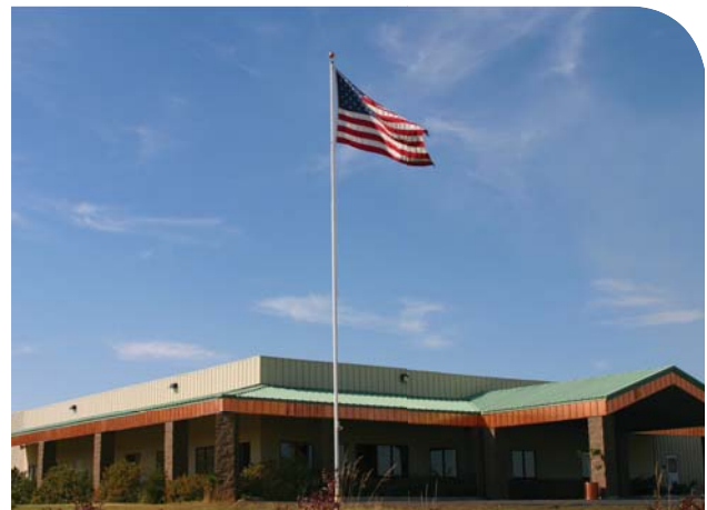
VMRD's facility is located in Pullman, Washington.
